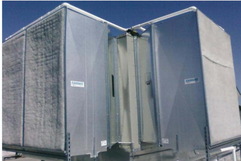
**Figure 2-1: AC#1 (LENNOX) with Bolt-On FlashCool Pre-Cooler**
