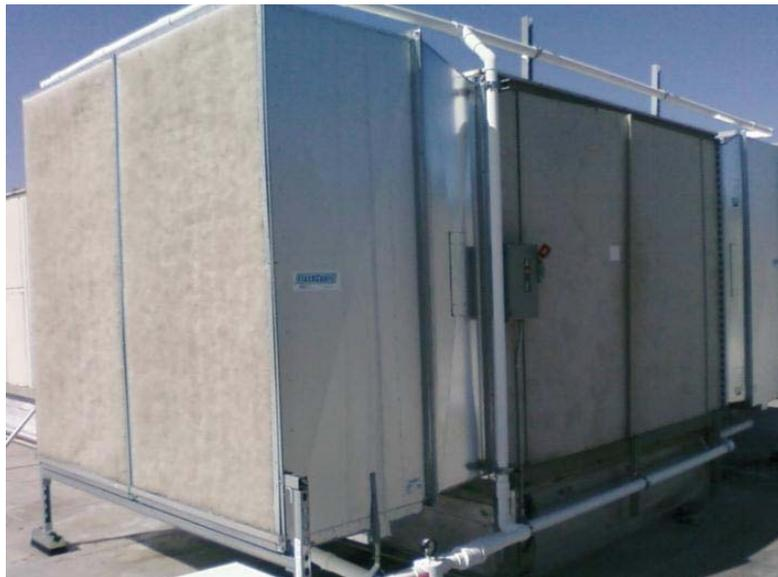
**Figure 2-2: AC#2 (TRANE) with Bolt-On FlashCool Pre-Cooler**
